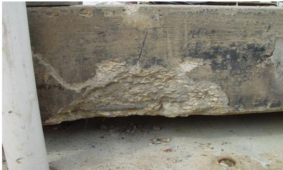
Figure 29: Carlisle Beam with Minor Evidence of Deterioration
