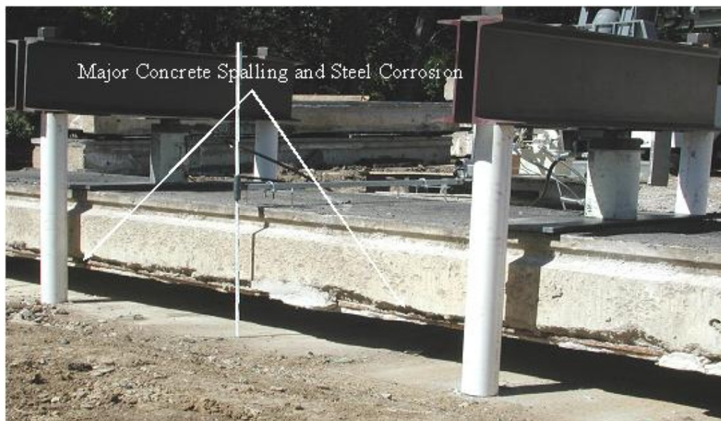
Figure 11: Precast Channel Beam in “Poor” Condition
