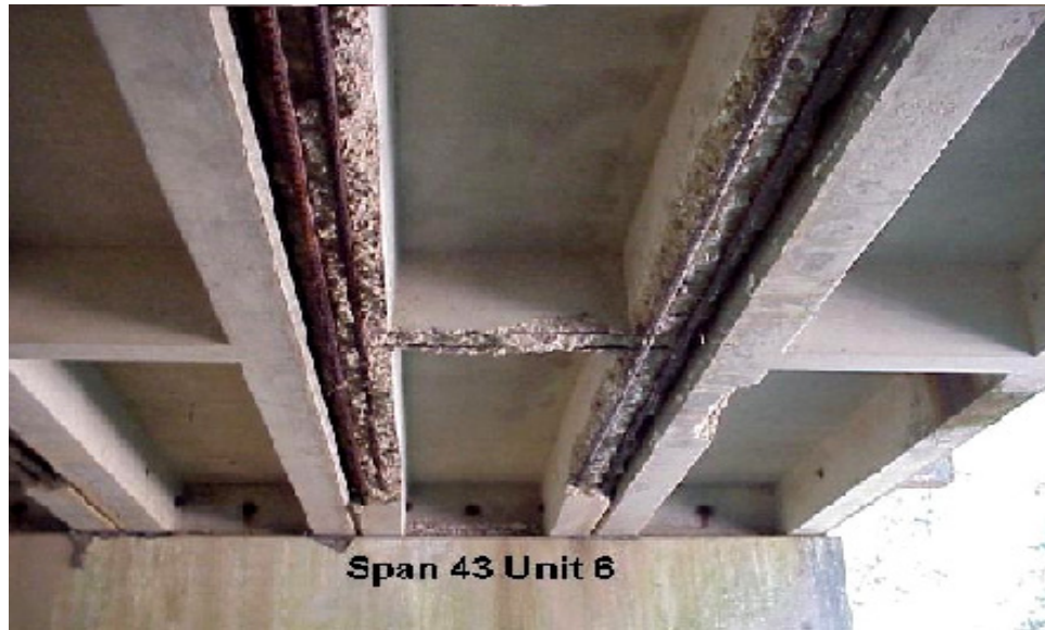
Figure 22: Concrete Spalling and Reinforcement Corrosion
