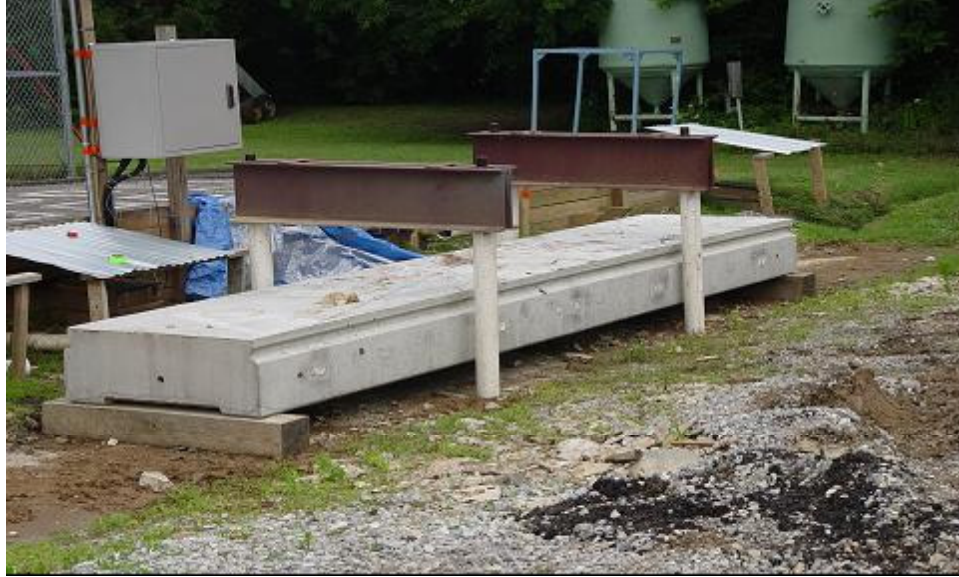
Figure 36: Newly Fabricated Channel Beam
