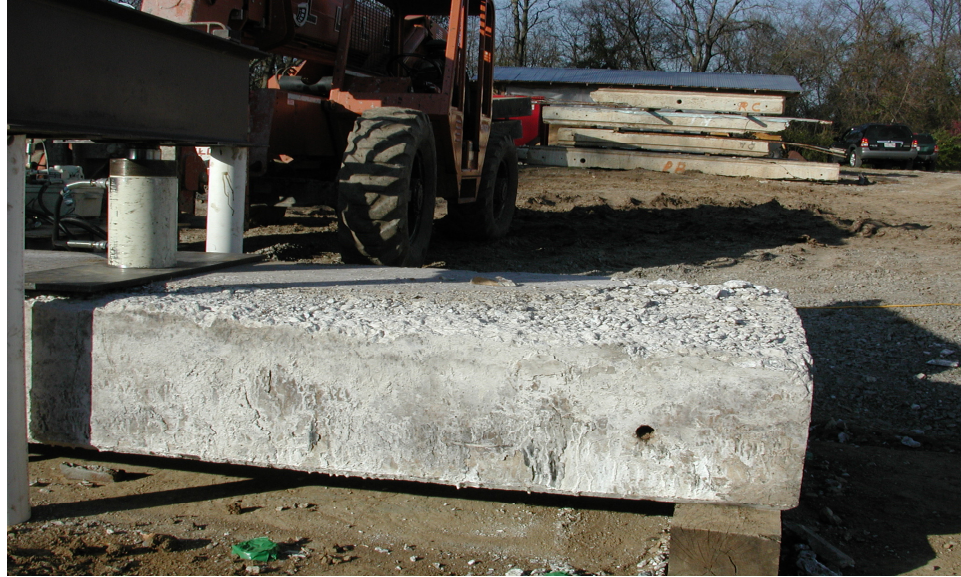
Figure 25: Poor Aggregate-Paste Bonding on Top of Beam
