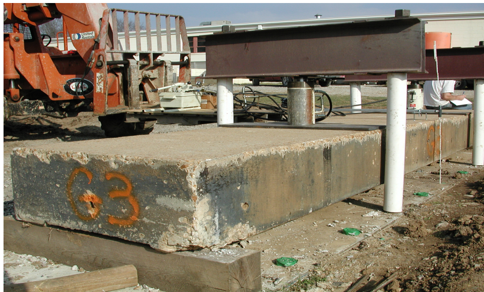
Figure 9: Precast Channel Beam in “Good” Condition
