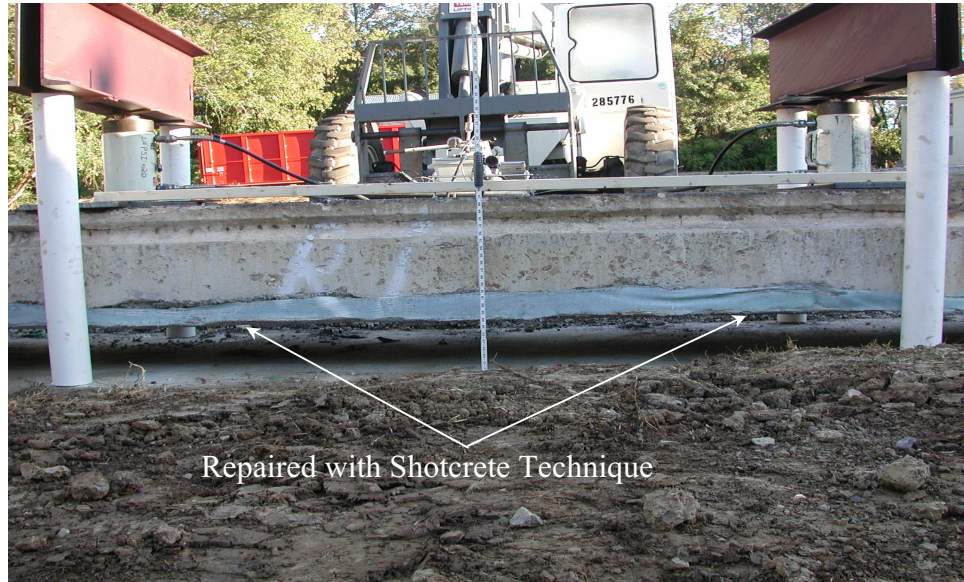
Figure 12: Precast Channel Beam in “Repaired” Condition
