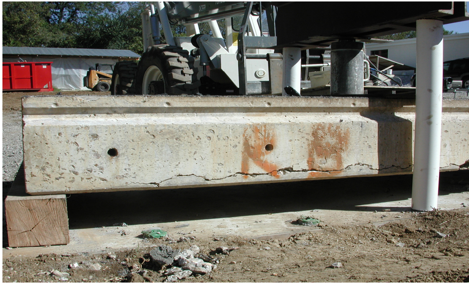
Figure 21: Longitudinal Cracking at the Height of the Reinforcement
