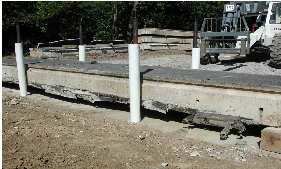
Figure 23: Shotcrete Technique Repair
