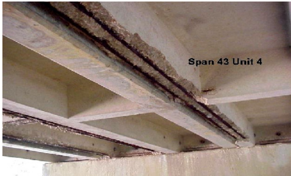
Figure 6: Deterioration of Jenkins' Ferry Bridge
