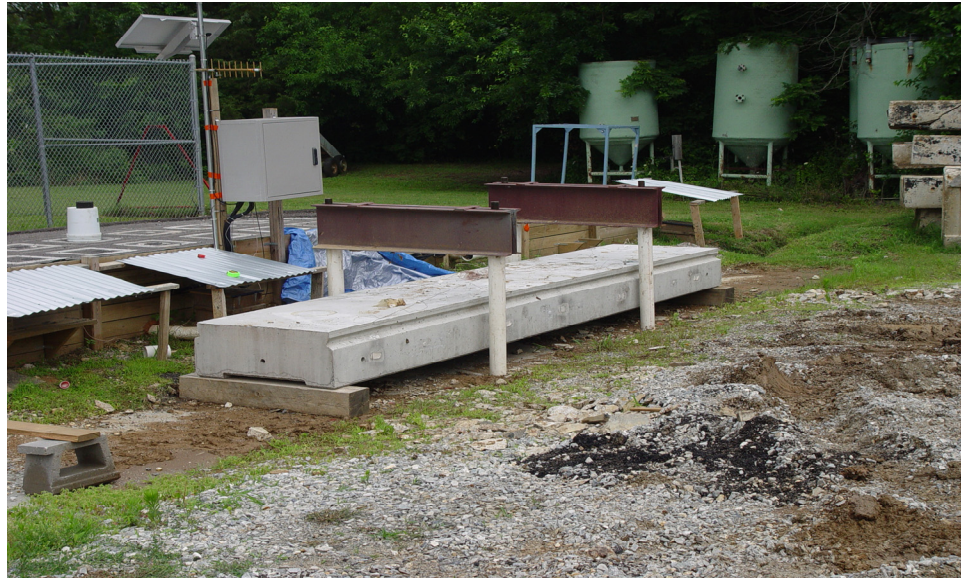
Figure 8: Precast Channel Beam in “New” Condition
