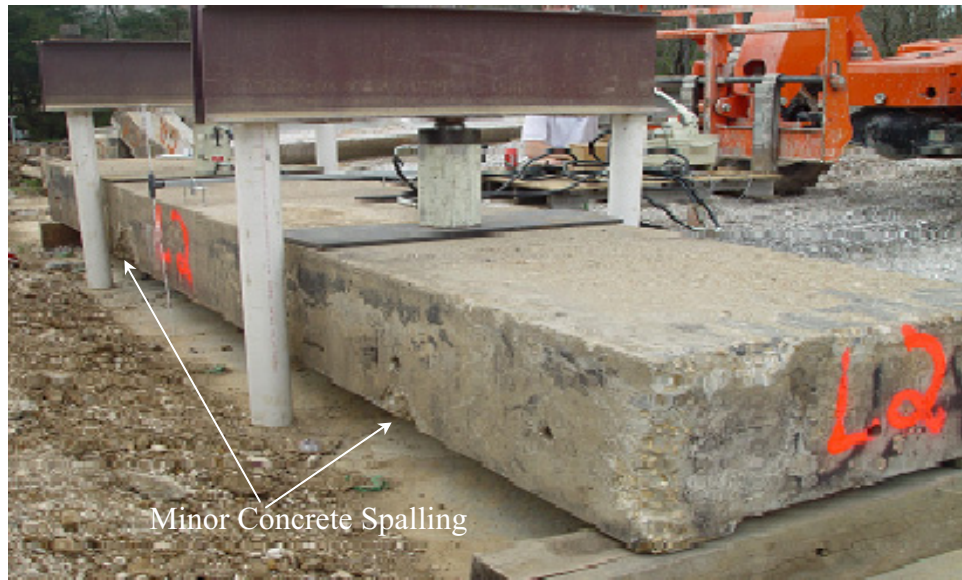
Figure 10: Precast Channel Beam in “Average” Condition
